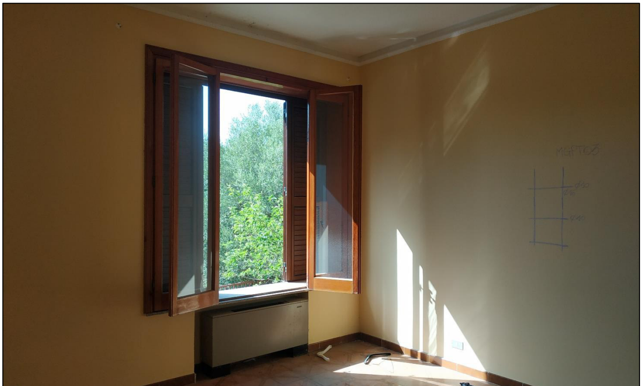
Figura 2-18 - Camera piano terra
