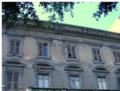
2. Palazzo Ex INAIL, Cagliari
