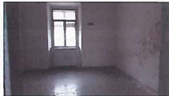
Interni – piano seminterrato
