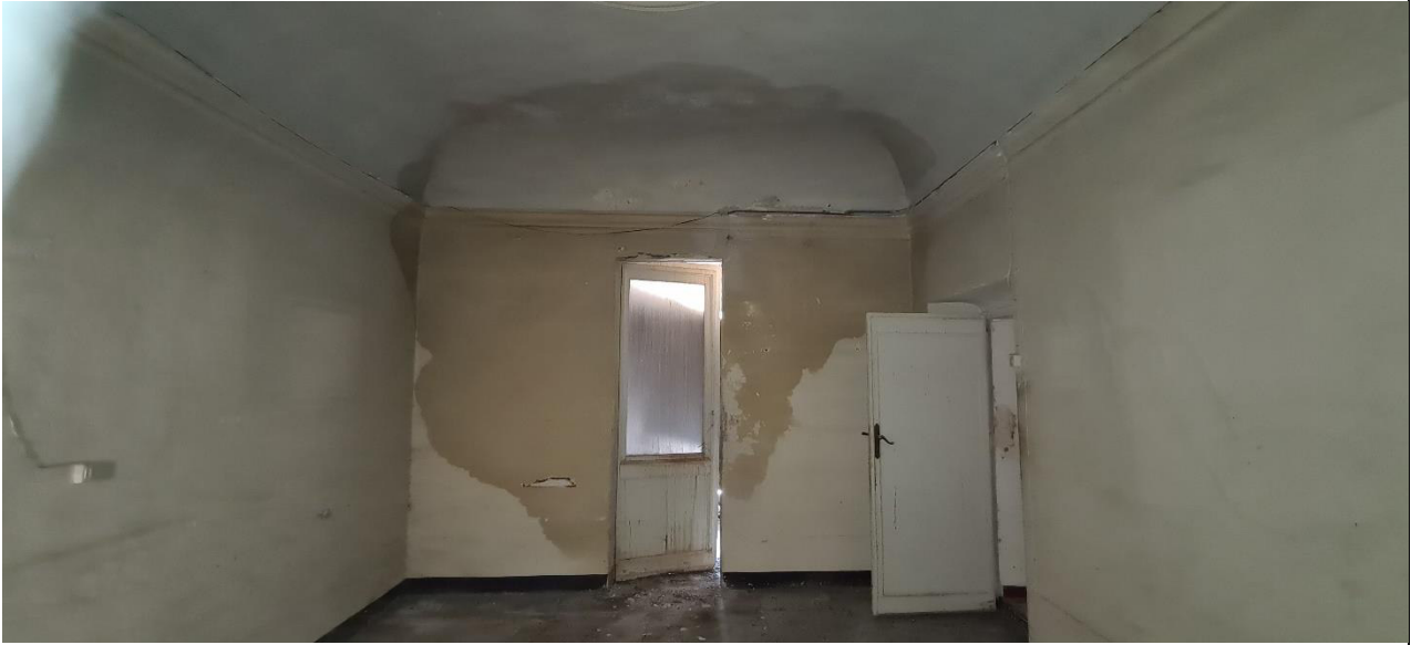
PARETE INTERNA PIANO TERRA
