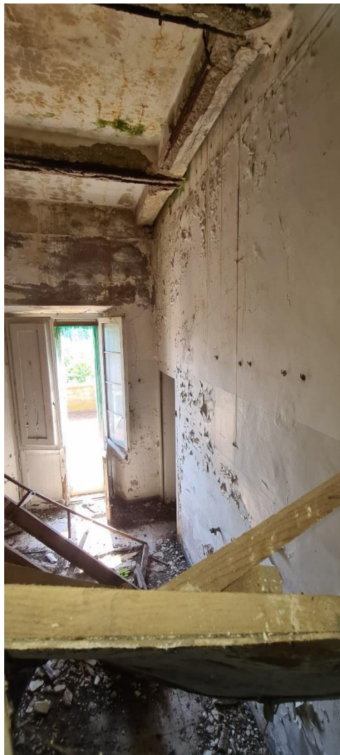
LOCALE PIANO TERRA
