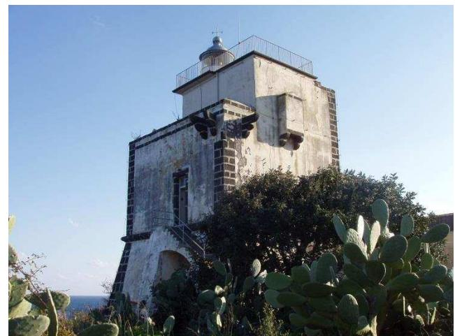
**Capo Mulini Lighthouse** is located close to the Town of Acireale, in the Gulf of Catania (in the eastern part of the Region of Sicily), in a truly remarkable panoramic context. The main building is a two-storey structure, built with lava stones at the corners with the light on the top of it. It is also contains the home of the former lighthouse keeper.
